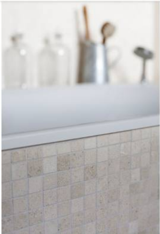
Natural stone, or stone effect porcelain tiling, 600x600mm on floor, 600x300mm on walls, 50x50mm mosaics for floor and wall detailing, 25x25mm on floor of shower enclosure.
