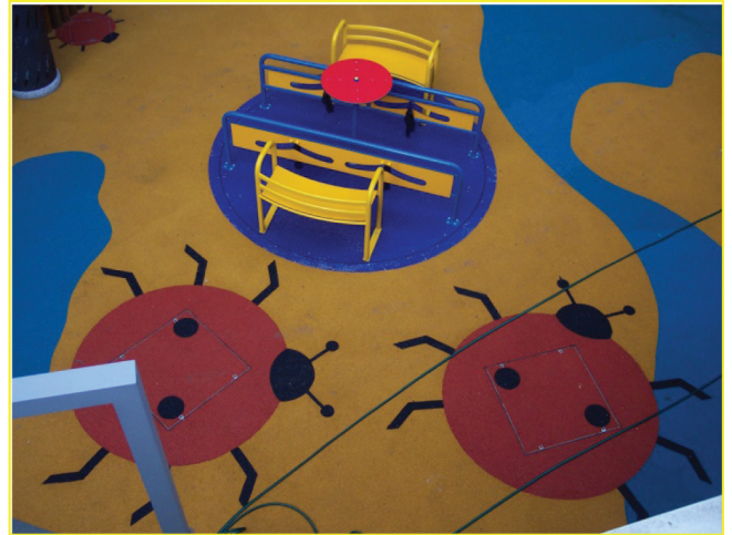
Continuous wet pour surfacing – with graphics
